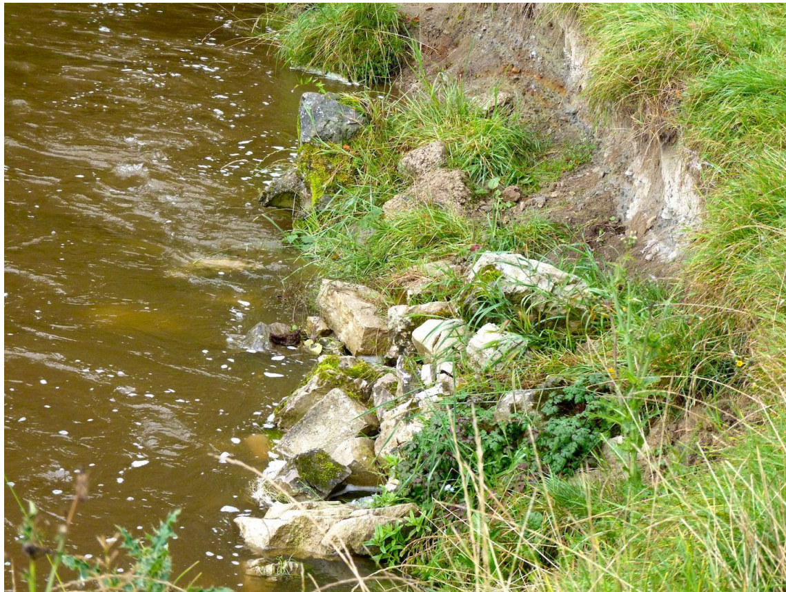
A river cliff on a meander that has had rocks placed near it to slow down erosion.
