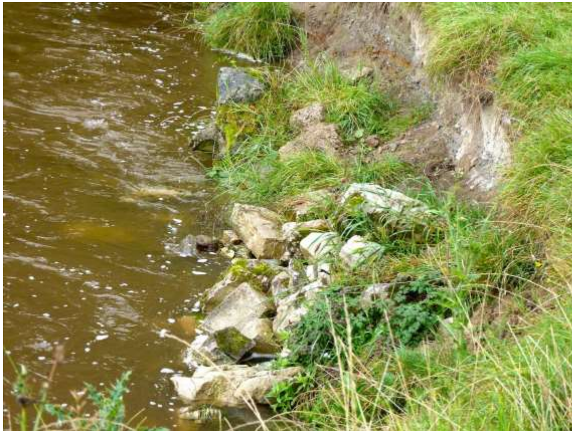
A river cliff on a meander that has had rocks placed near it to slow down erosion.
