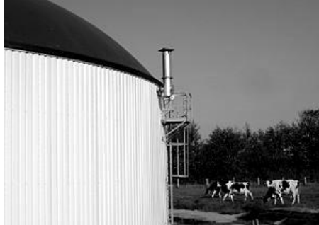
Anaerobic digesters for silage
