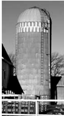
Concrete silage silo
