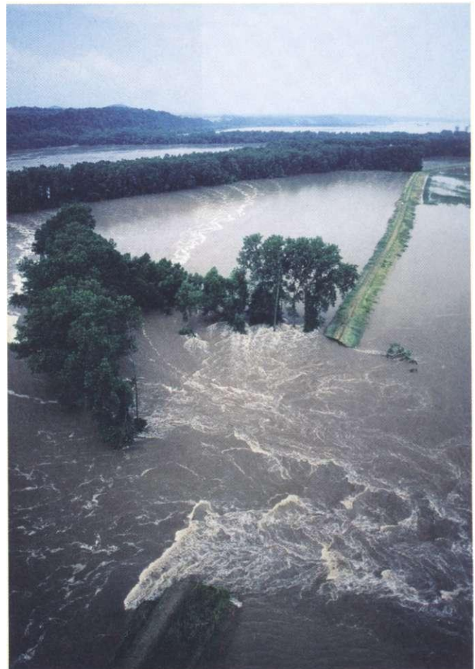
Figure 8.3 Levee failure Failure of this levee in Illinois during the 1993 floods of the Mississippi River caused flooding in the town of Valmeyer. (Comstock Images)
