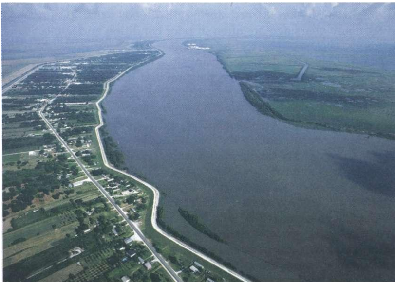
Figure 8.24 Mississippi River levee A levee with a road on top of it protects the bank (left side of photograph) of the lower Mississippi River at this location in Louisiana. (Comstock Images)
