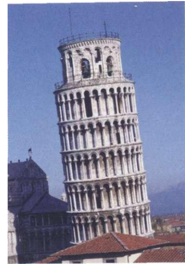
Figure 16.8 Leaning Tower of Pisa, Italy The lean is a result of differential settling of the soil. If correction measures had not been taken to strengthen the tower, it would have fallen over. (D. & J. Heaton/Stock Boston)
